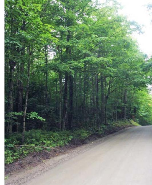
**ABOVE LEFT** *Roadside ditch construction created a bare backslope prone to erosion. Road crews can consider reducing the angle of the backslope, hydroseeding the bare soil, or planting live stakes in the backslope to reduce soil erosion. Outsloping the road so that runoff flows into vegetation downhill will also reduce the need for ditching on the upslope side and help preserve trees.*
