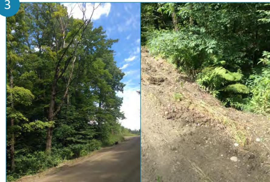
Damage to trees, shrubs and grasses may be the result of both roadwork and erosion along Garfield Road. Consider the connection of this road to the downslope stream and how both road reinforcements and planting could protect this roadside.
