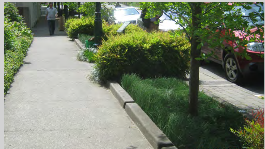
▲ These street stormwater planters have no side slope condition and have only one planting zone featuring wet-tolerant plant material.
