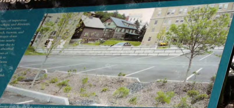
Stormwater runoff in a parking lot at 133 State Street captures and treats stormwater runoff. Credit: Vermont Department of Buildings & General Services.
