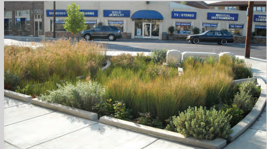
▲ This street rain garden has two planting zones with dry-tolerant plants placed on the side slopes and wet-tolerant plants placed at the lowest elevations..
