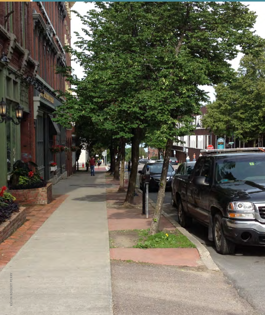
BURLINGTON, VERMONT: Driveway curb cuts and narrow storefront sidewalks.
