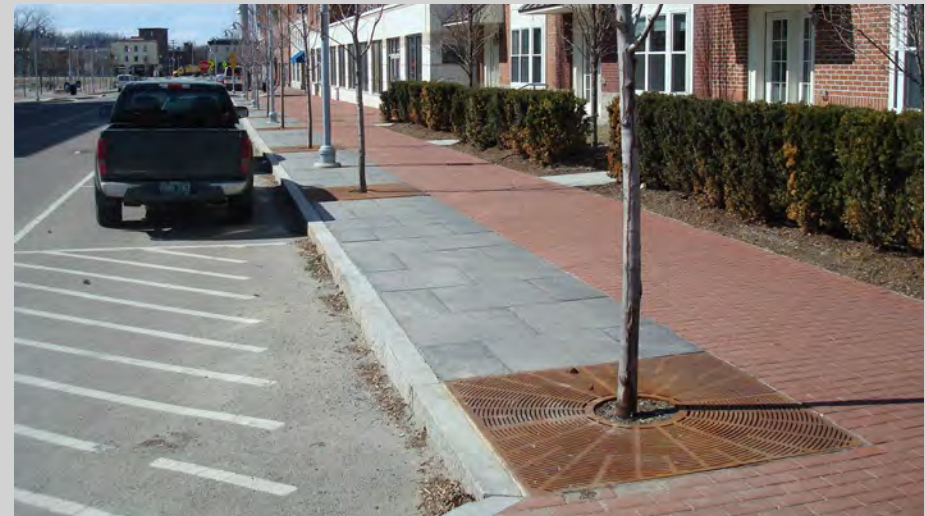
▲ These street trees are installed with structural soil to increase soil volume and allow for greater root expansion. (Winooski)
