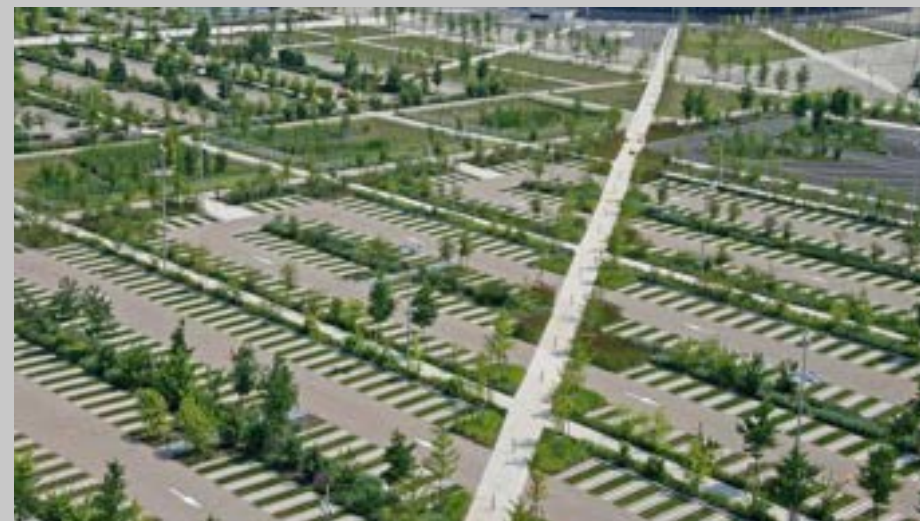
▲ This parking lot example in France significantly increases pervious surfaces and landscaping within the parking lot, provides for safe pedestrian circulation, and manages runoff on site.
