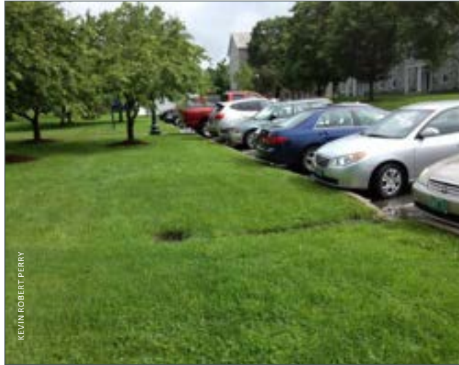
▲ Existing lawn areas can be transformed into rain gardens that capture and treat runoff prior to entering the storm drain system.
