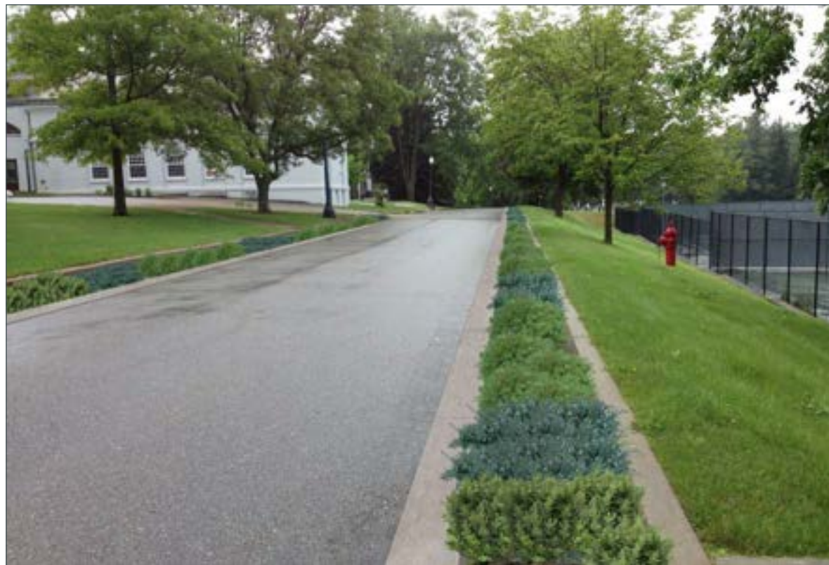
▲ RETROFIT OPPORTUNITY: The same residential street retrofitted with a green gutter. In this example, the green gutter is only within the street leaving the existing curb in place and replaces the failing asphalt area.
