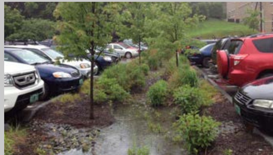
▲ Green Streets captures runoff and pollutants and treats it prior to entering a nearby creek, stream, river, or lake. (Montpelier, VT)
