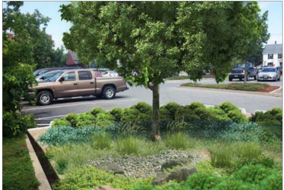
▲ RETROFIT OPPORTUNITY: The same parking lot in Middlebury, VT retrofitted with a stormwater planter replacing two parking stalls near the existing drain inlet.
