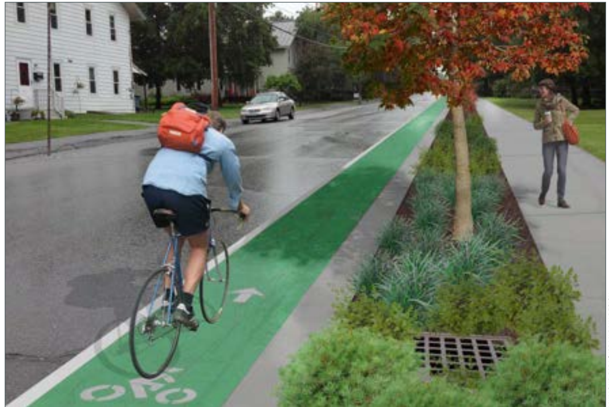
▲ RETROFIT OPPORTUNITY: The same residential street retrofitted with a vegetated swale, optional bike lane, as well as additional street trees. In this example, the vegetated swale helps separate the sidewalk zone from vehicular traffic.
