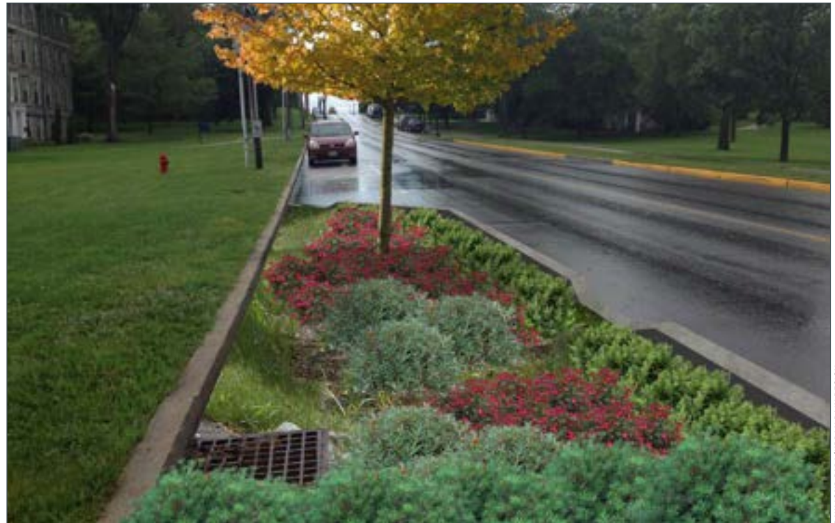
▲ RETROFIT OPPORTUNITY: The same residential street retrofitted with stormwater curb extensions, as well as additional street trees. In this example, the curb extension is only within the street leaving the existing curb in place.
