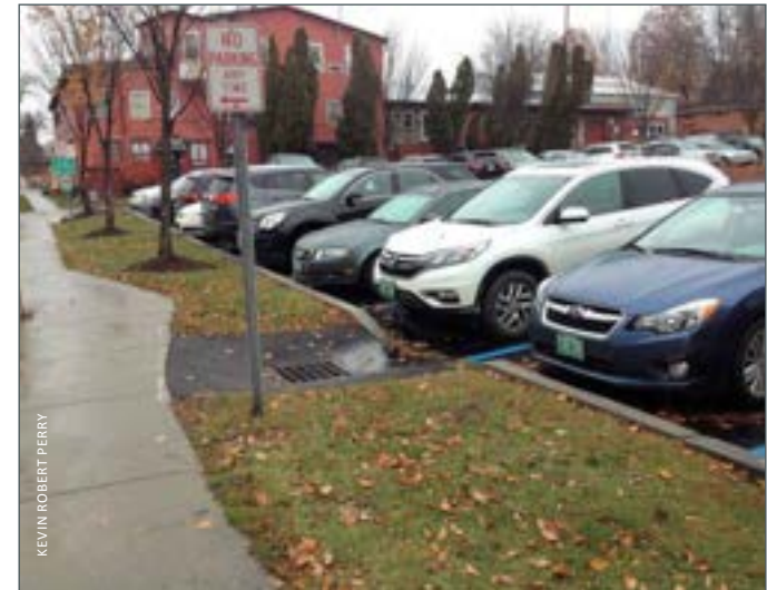
▲ Even well-used parking lots sometimes have existing landscaped space that can be redesigned to capture runoff.
