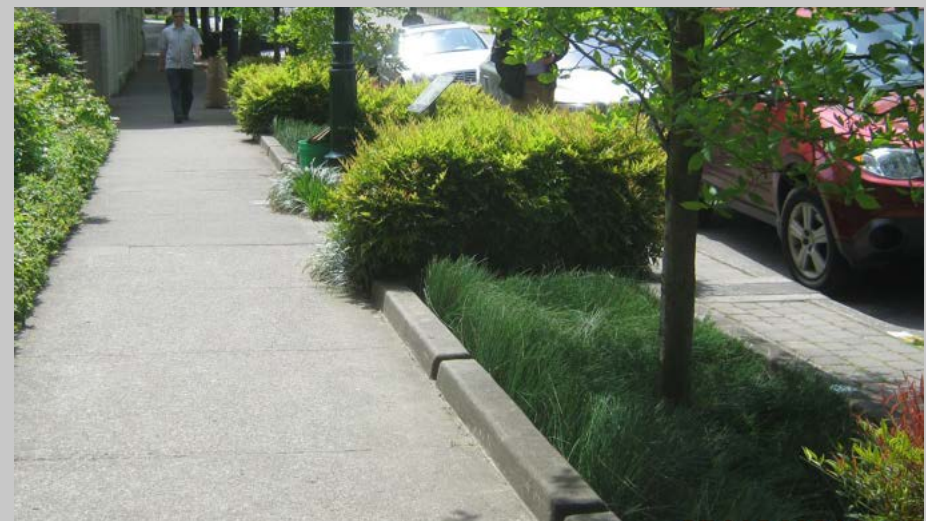
▲ These street stormwater planters have no side slope condition and have only one planting zone featuring wet-tolerant plant material.
