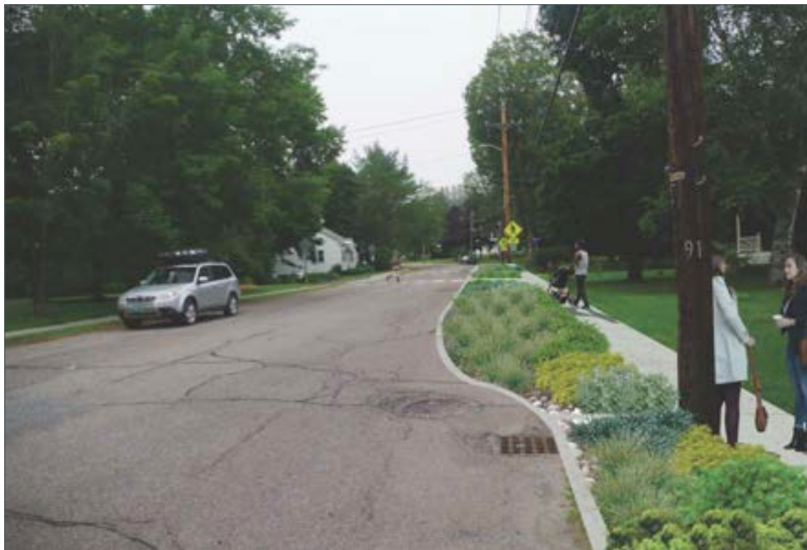
▲ RETROFIT OPPORTUNITY: The same residential street retrofitted with staggered mid-block stormwater curb extensions. Take note that the staggered condition helps create a traffic calming feature.
