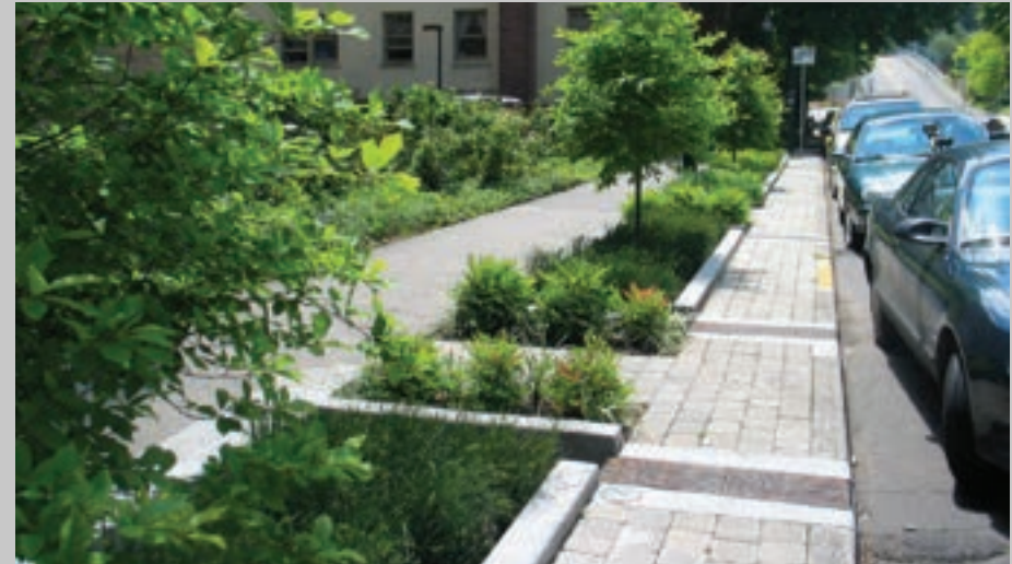
▲ This Green Street project utilizes a series of stormwater planters while maintaining on-street parking and adequate space for pedestrian circulation.
