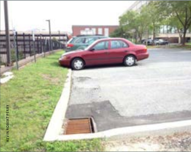
▲ Parking stalls that are not heavily utilized can be converted into landscaped areas designed to capture runoff
