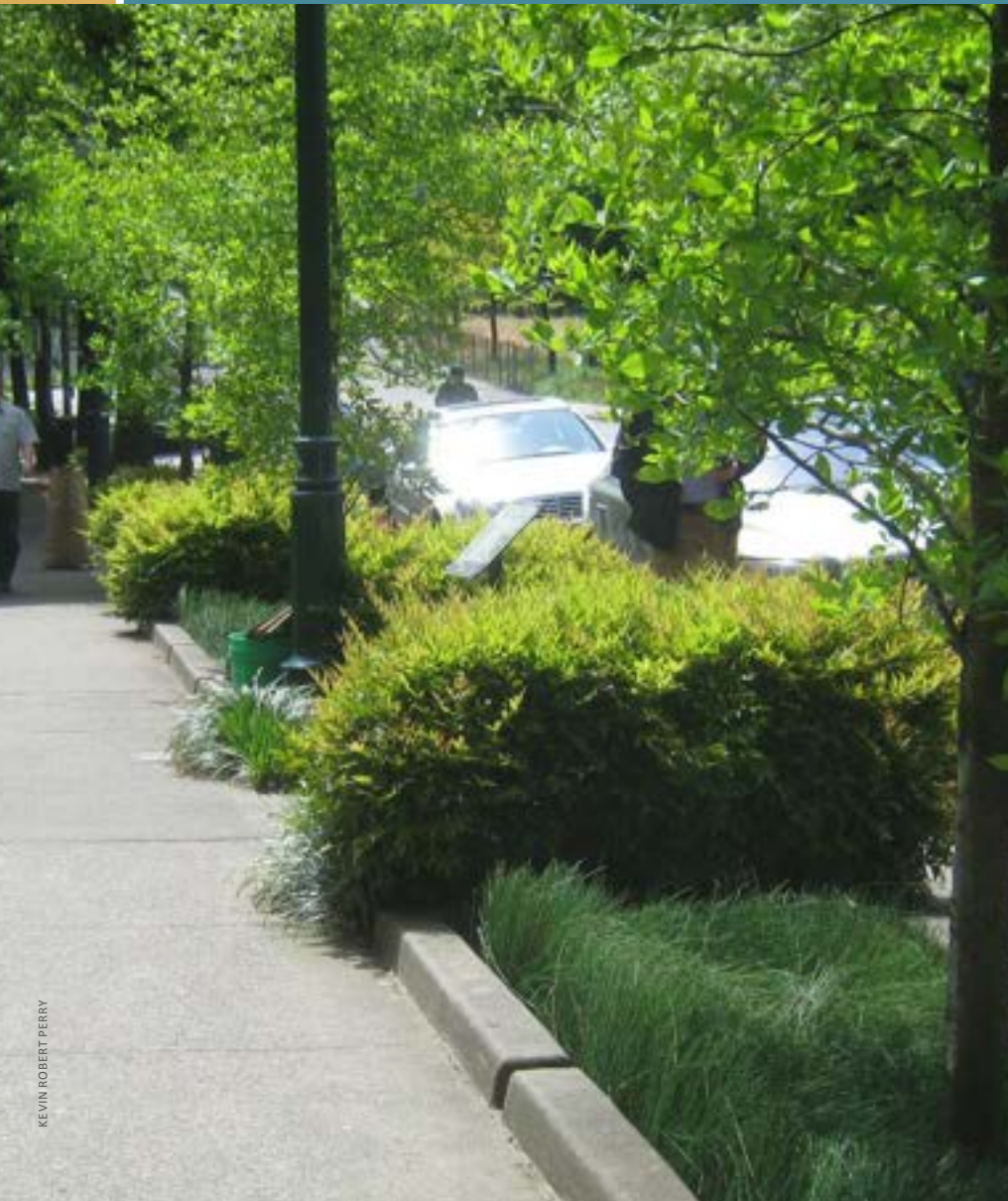
PORTLAND, OREGON: Stormwater planters along SW 12th Avenue.
