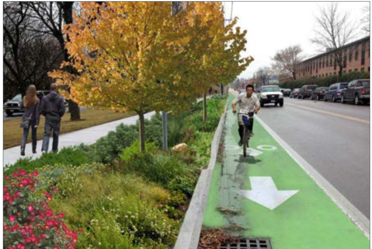
▲ RETROFIT OPPORTUNITY: The same arterial street retrofitted with a vegetated swale, as well as additional street trees. In this example, the vegetated swale only is within the existing landscape strip leaving the existing curb in place.
