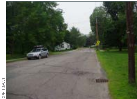
▲ EXISTING: A typical low-density residential street in Vermont.
