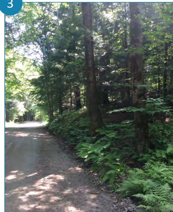
An example of a roadside forest dominated by mature ( > 6 " DBH) overstory trees in the right-of-way. Also present is an established understory.
