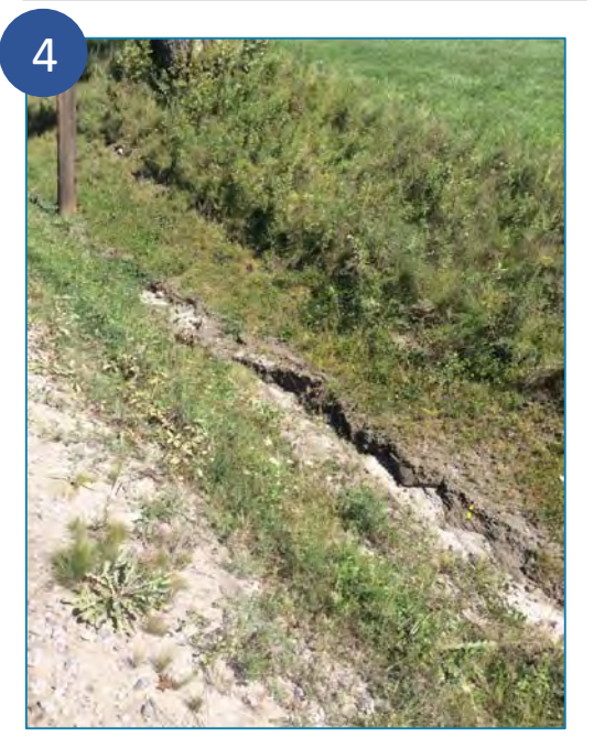
4 The utility pole is now located in a shallow roadside ditch along Hollister Hill Road. Consider revegetating the area surrounding the utility pole to reduce the erosive power of stormwater runoff and to reestablish a buffer between the road and utility pole.
