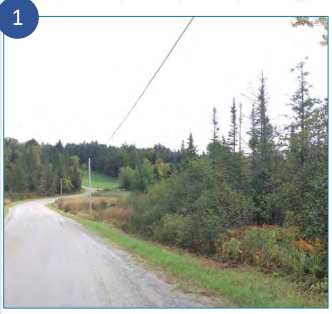
1 A 10-foot wide mowed zone next to the travelled portion of Beaver Meadow road keeps vegetation away from the utility line. However, the road and utility corridor passes directly through a wetland and pond. Examine why the mowed zone is wide here and if the utility company can do more to promote regeneration and preserve herbaceous buffer between the road and water body.
