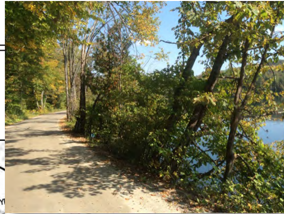
East side of Number 10 Pond Road north of GAR Road and parking area.
